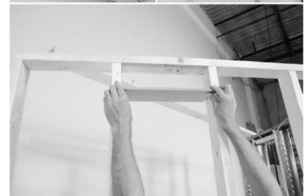
Use the "Go" gauge to verify that the minimum width of 14 3/8-inches is maintained over entire wall cavity height.
