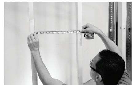
Use a tape measure to verify that the maximum width of 14 7/8-inches over entire wall cavity height is not exceeded.
