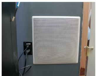
alignment and placement are so important that JL makes three different grille models, with depths to fit wallboards ranging from a half-inch to 1.9/16 inches thick.
